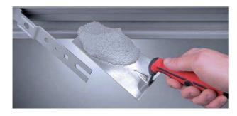
For mortar fixing, appropriate cuts will need to be created in the walls (section 80 x 200 mm). The anchors should be bent and blocked inside the wall. For fire sealing purposes and a perfect mechanical fit, the space between the doorframe and the masonry shall always be filled with concrete mortar.
