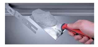
For mortar fixing, appropriate cuts will need to be created in the walls (section 80 x 200 mm). The anchors should be bent and blocked inside the wall. For fire sealing purposes and a perfect mechanical fit, the space between the doorframe and the masonry shall always be filled with concrete mortar.
