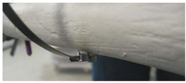
2. Tense the band with the tensioner and the torque screwdriver.
